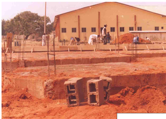
Construction of research library, Gombe Federal College
