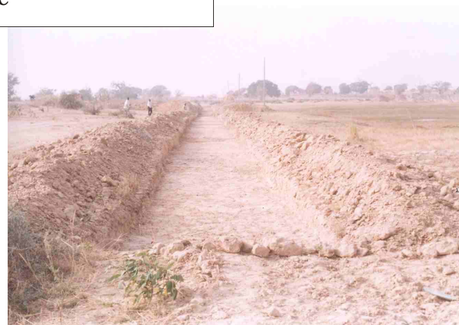
Construction of water harvesting structures, Dutse
