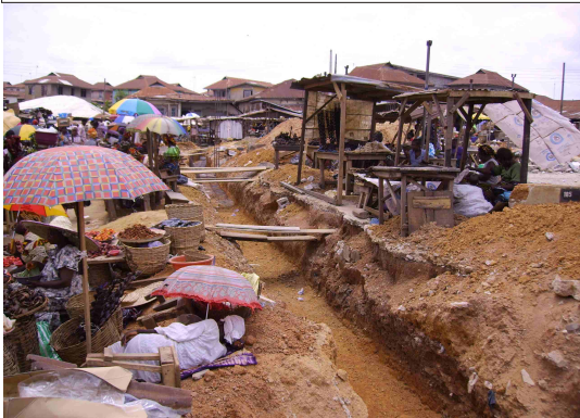
Improved drainage, Showing before (left) and after (right)
