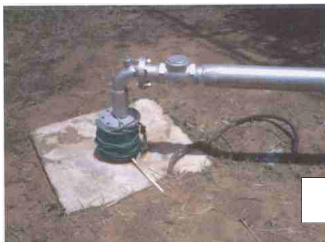
Borehole headworks
