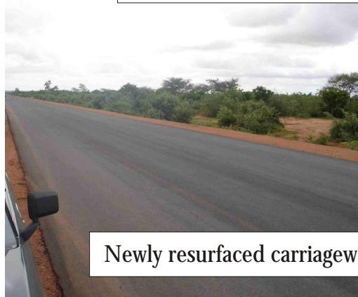
Rehabilitation of Funtua-Sokoto-Gusau Road
